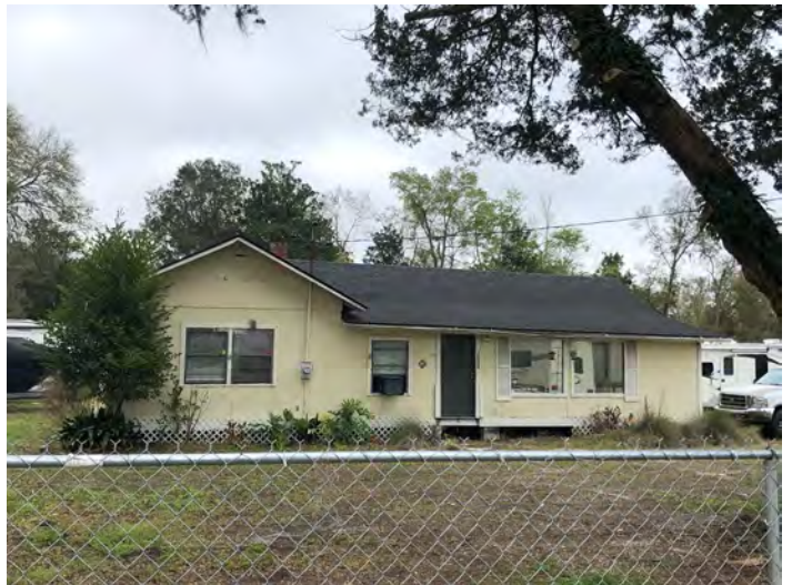
8DU16143_d Facing East
