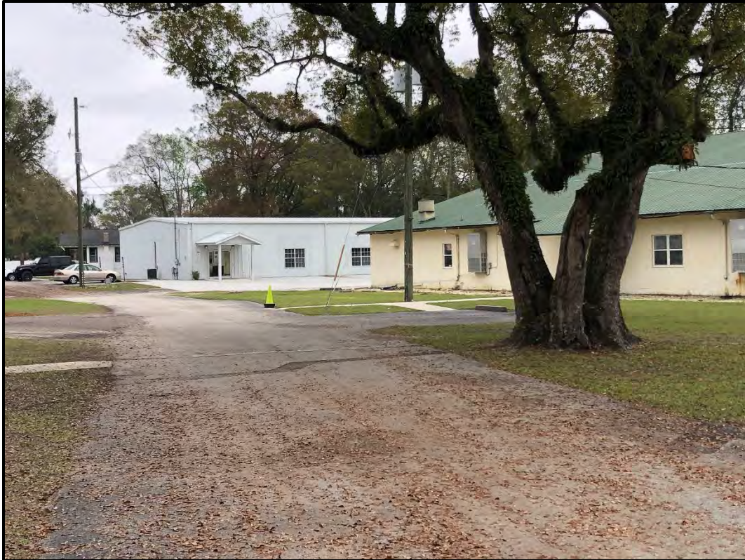
Location of demolished Resources 8DU016144-8DU16146, facing east.
