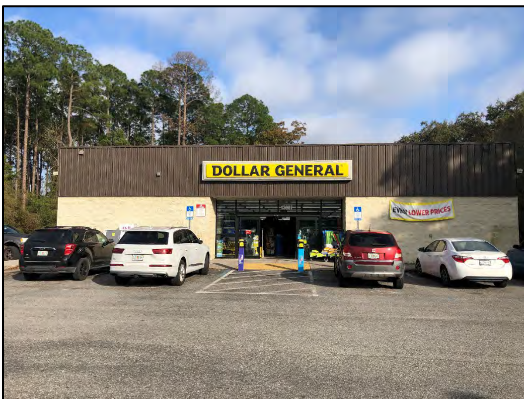
Location of demolished Resource 8DU16140, photograph facing east.
