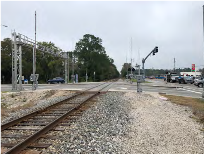
8DU21308_a Facing North
